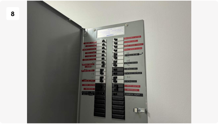
Project: Common Area Date: Sep 16, 2025, 1:42 PM Creator: Adam Clements
