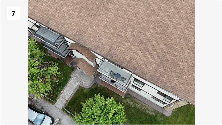
Project: Exterior Date: Sep 16, 2025, 12:43 PM Creator: Adam Clements
