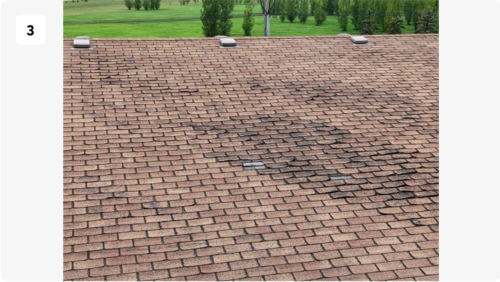
Project: Exterior Date: Sep 16, 2025, 12:40 PM Creator: Adam Clements
