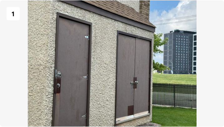
Project: Electrical Room Date: Sep 16, 2025, 1:50 PM Creator: Adam Clements
