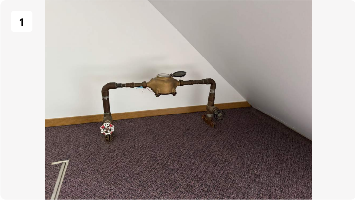
Project: Common Area Date: Sep 16, 2025, 1:00 PM Creator: Adam Clements
