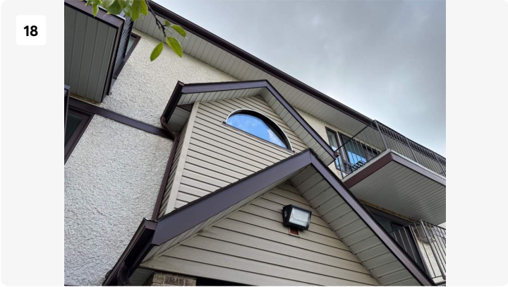
Project: Exterior Date: Sep 16, 2025, 1:54 PM Creator: Adam Clements
