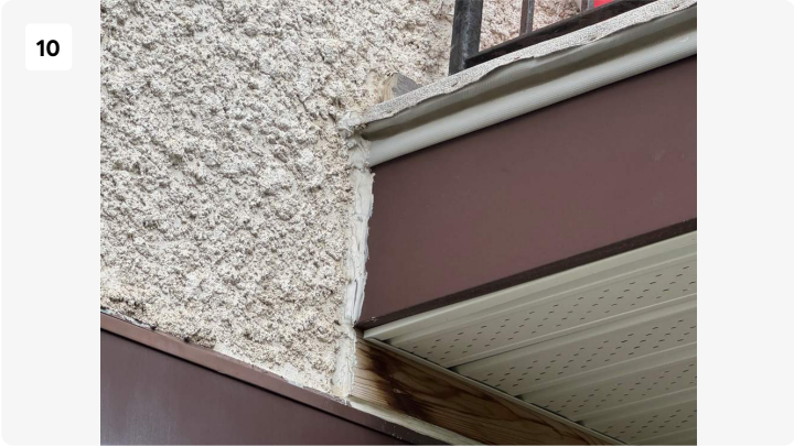
Project: Exterior Date: Sep 16, 2025, 12:54 PM Creator: Adam Clements
