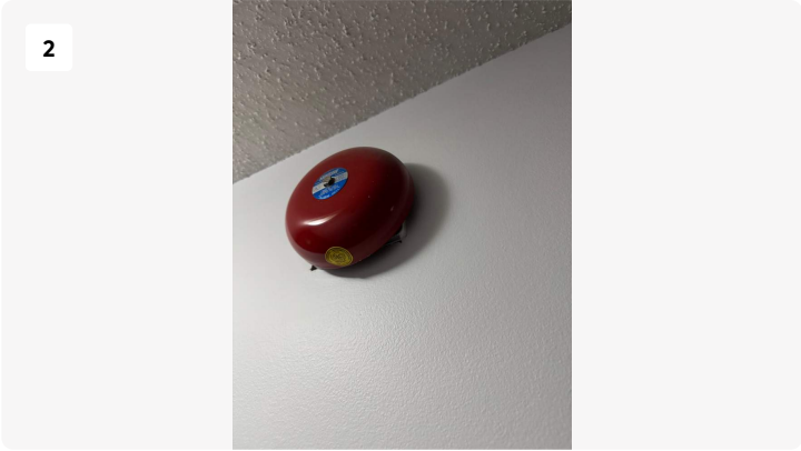
Project: Common Area Date: Sep 16, 2025, 1:17 PM Creator: Adam Clements
