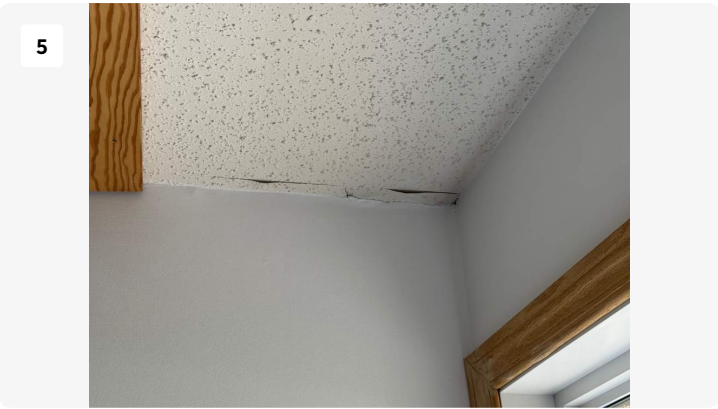
Project: Common Area Date: Sep 16, 2025, 1:19 PM Creator: Adam Clements
