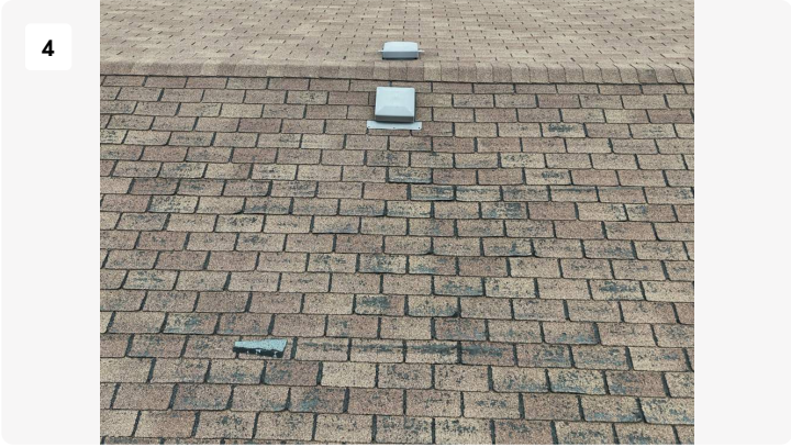
Project: Exterior Date: Sep 16, 2025, 12:41 PM Creator: Adam Clements
