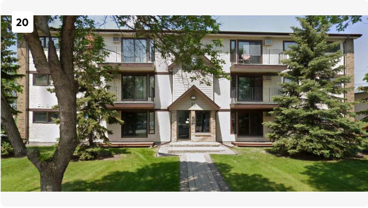
Project: Exterior Date: Sep 28, 2025, 11:28 PM Creator: Adam Clements
