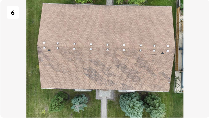
Project: Exterior Date: Sep 16, 2025, 12:42 PM Creator: Adam Clements
