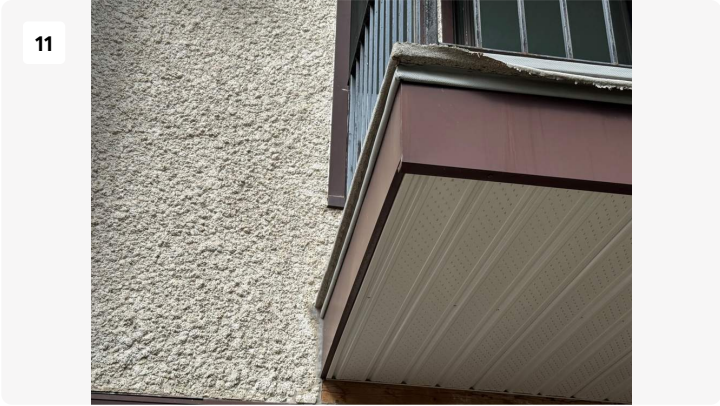
Project: Exterior Date: Sep 16, 2025, 1:49 PM Creator: Adam Clements
