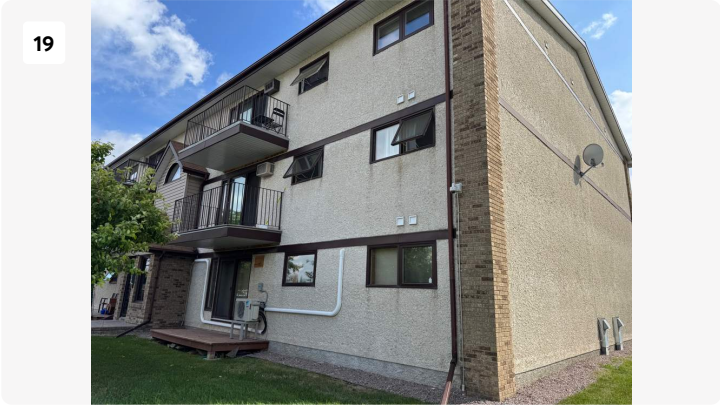
Project: Exterior Date: Sep 16, 2025, 1:55 PM Creator: Adam Clements
